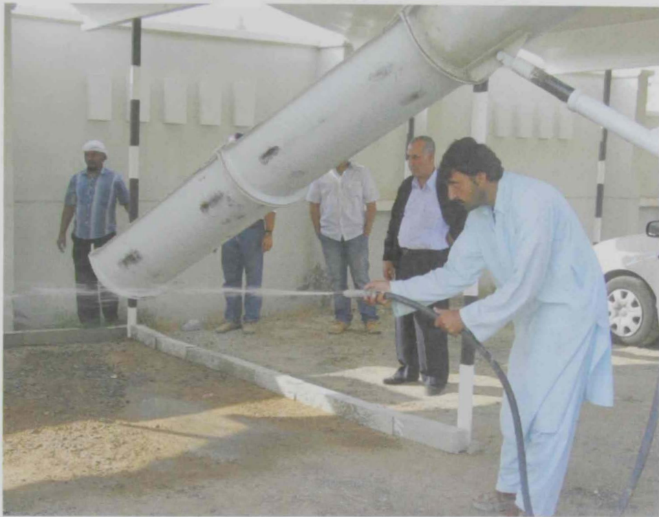
Figure 6: Wash down the concrete truck chute by water
