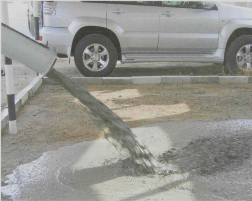
Figure 7: The poured concrete was used in paving a parking lot
